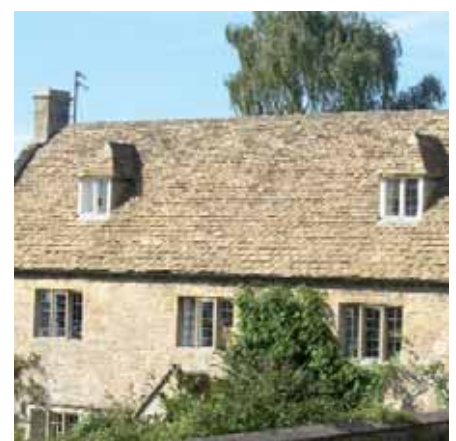
Large buildings contrast with modest cottages giving a pleasing variation in character
