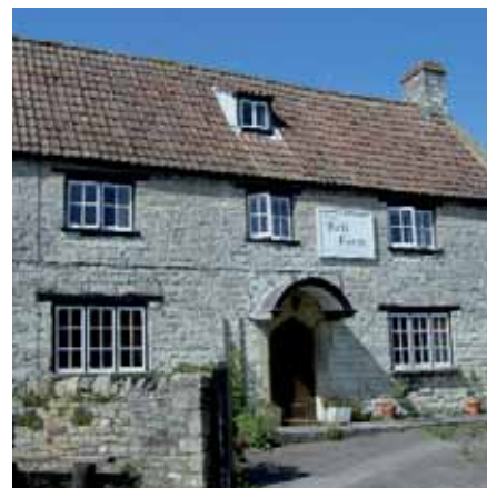
Most of the buildings are built from the local lias stone which creates a distinct sense of place
