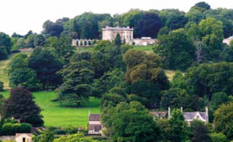
View from across the valley
