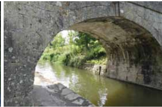
Ferry Lane Bridge
