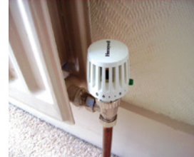
Install heating controls
