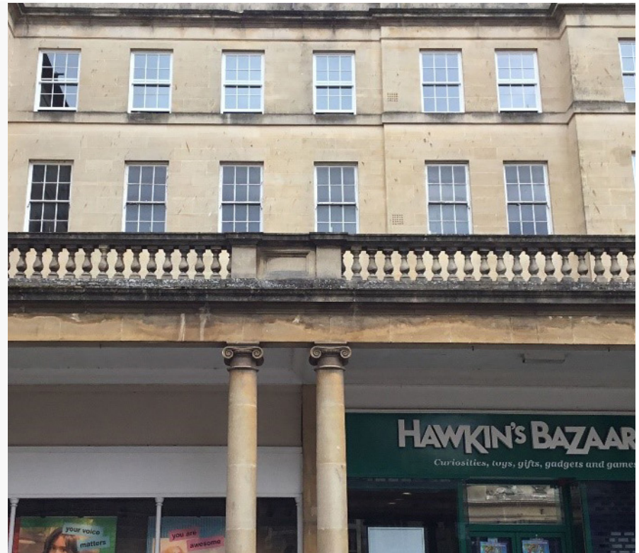
Replacement slimline (12mm) double-glazed sash windows alongside existing original single-glazed windows in Arlington House, Stall Street, Bath.
