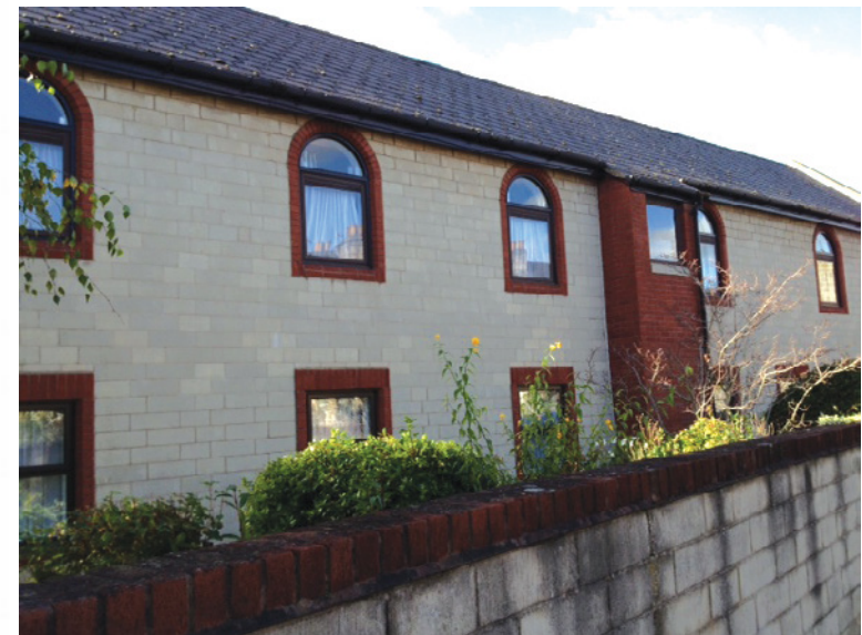
Example of a Late 20 th Century Building in Bath & North East Somerset
