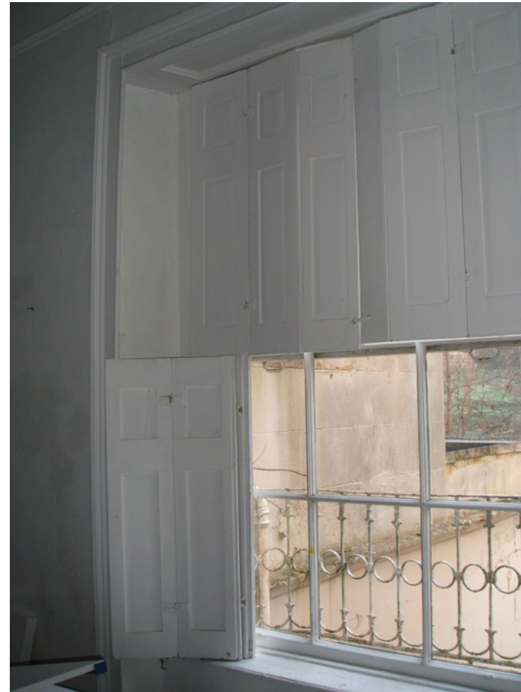
Existing shutters at Somerset Place, Bath
