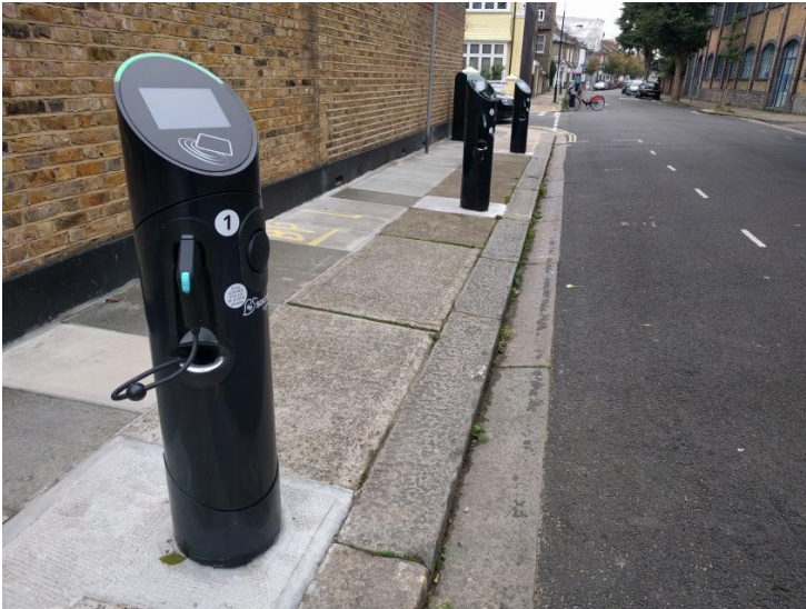
Figure B-2: Floor mounted bollard charging point
