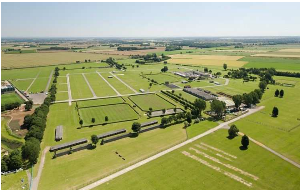
Figure 5-3 - Temporary Park and Ride in Lincoln
