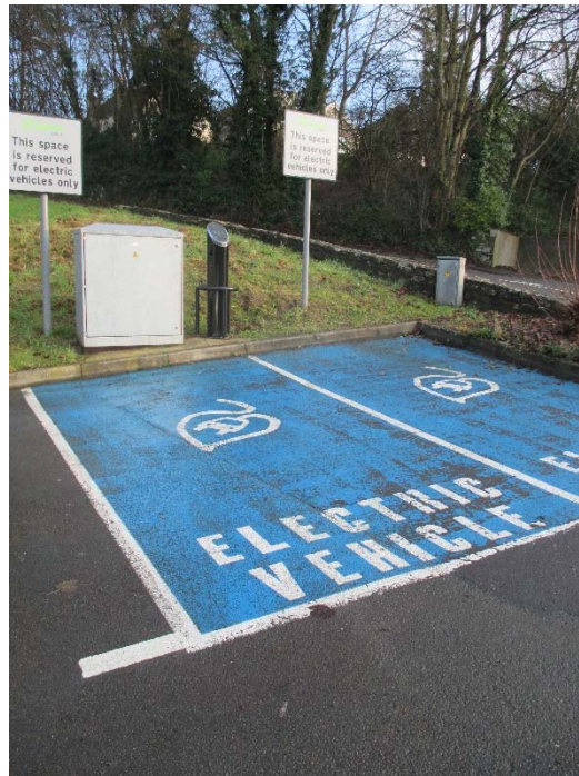
Figure 8-1 Electric Charging Point Spaces at Fox and Hounds Car Park, Keynsham
