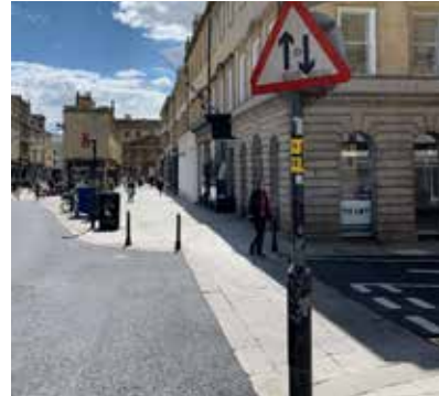
Pedestrian priority causeways over Quiet Street at Milsom Street junction
