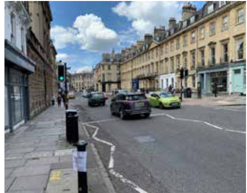
Signal controlled crossing on George Street
