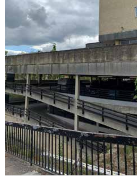
Podium multi-storey car park adjacent to the River Avon
