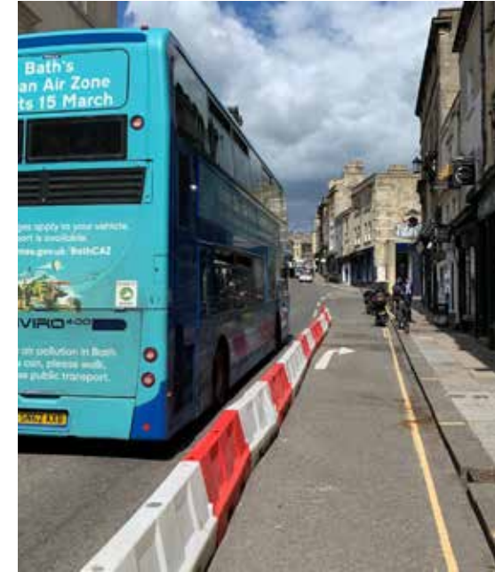
Northbound bus passing temporary footway widening on Broad Street
