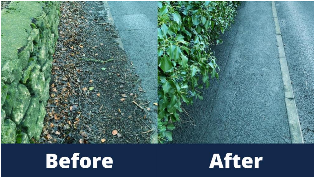
Weeds and leaves removed along Claverton Down Road, Combe Down
