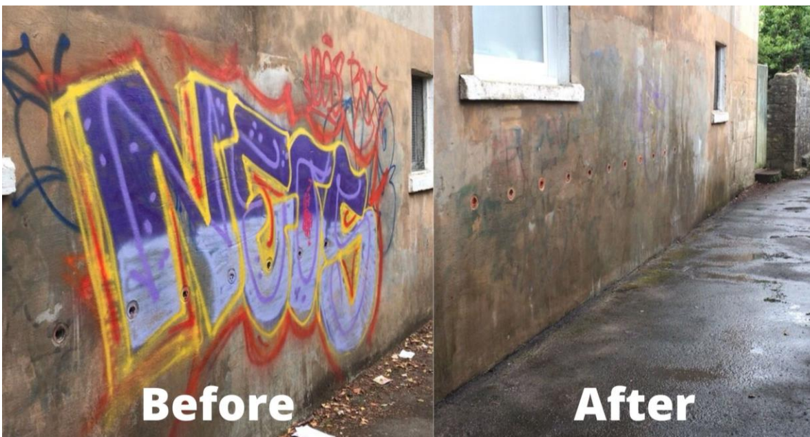
Graffiti removed from a domestic property on Bradford Road, Combe Down
