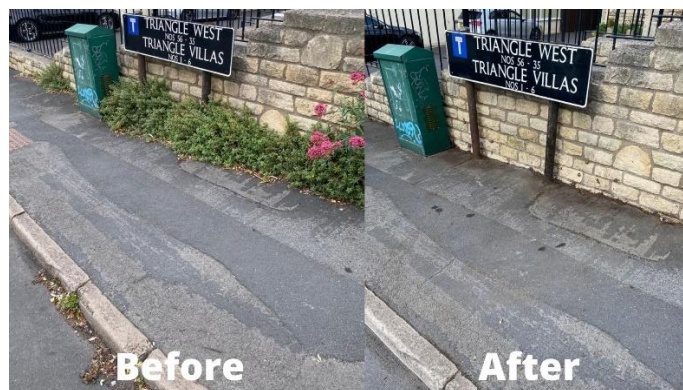
Weeding and sweeping completed along Triangle West, Westmoreland
