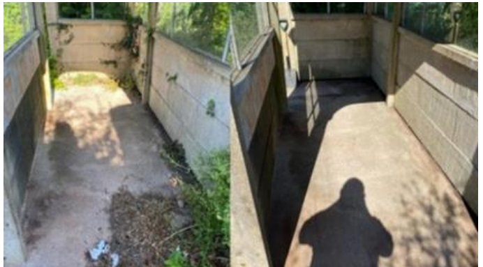
Sweeping and weed removal completed from bus shelter on The Crescent, High Littleton
