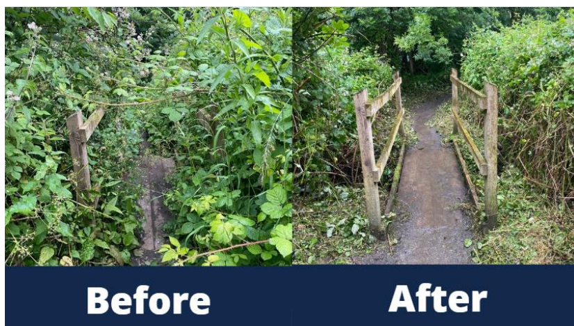
Vegetation removal at the Archery Fields, Weston Park West, Weston.
