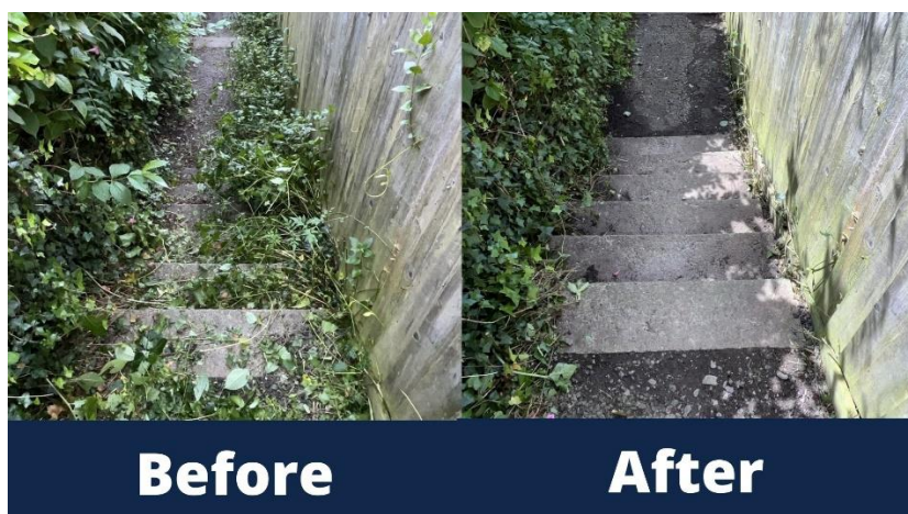
Vegetation removal at Purlewent Drive, Laneway, Weston.
