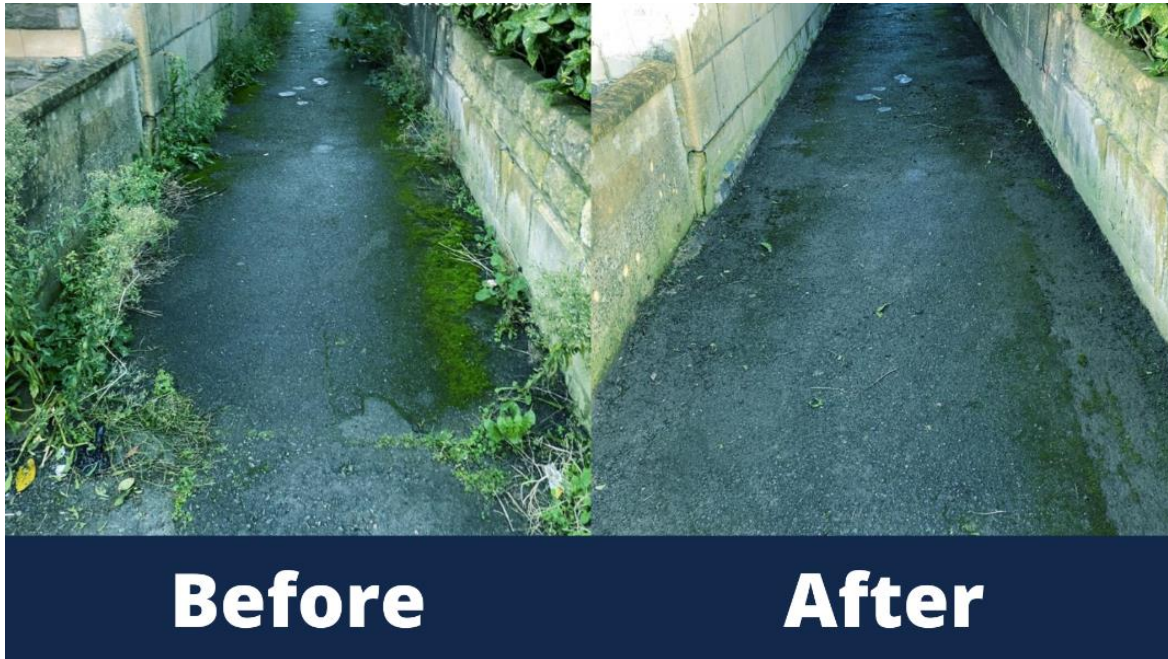
Weeds cleared along laneway at Third Avenue in Oldfield Park
