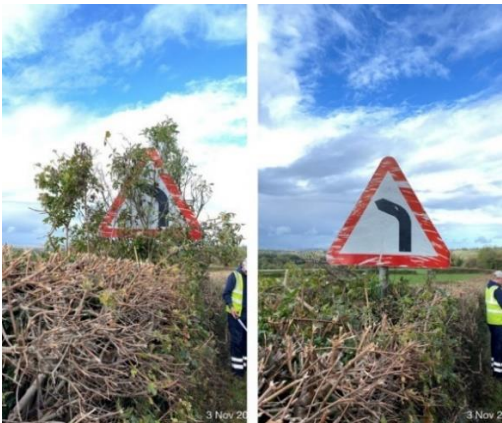
Overgrown vegetation removed on Bath Road, Newbridge
