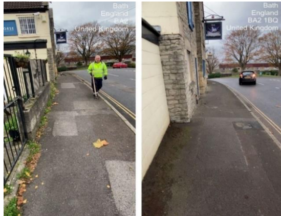
Sweeping and weed removal completed along Shophouse Road, Twerton
