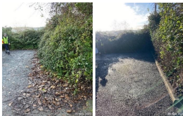
Overgrown vegetation removed on Green Tree Road, Midsomer Norton
