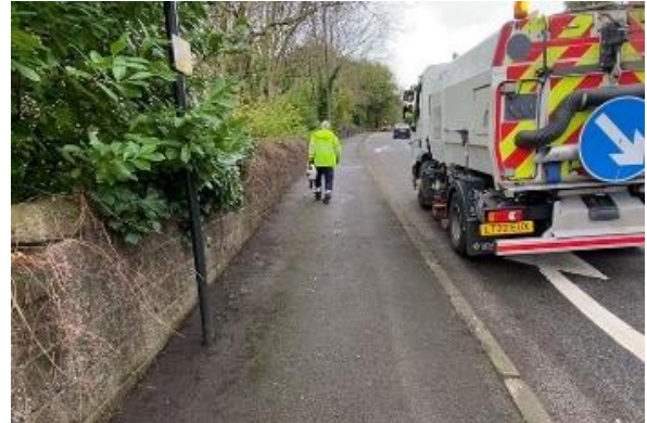
Sweeping and weed removal completed along Wellsway Road, Widcombe and Lyncombe
