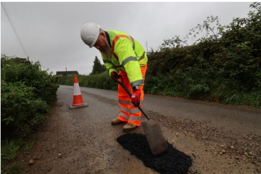
Highway Inspector repairing pothole in Upton Lane, Chew Magna
