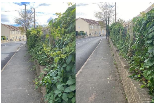
Overhanging vegetation cut back along Bristol Road, Whitchurch
