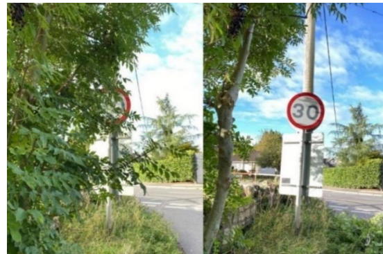
Before and after picture of overgrown vegetation blocking a sign removed in Farmborough
