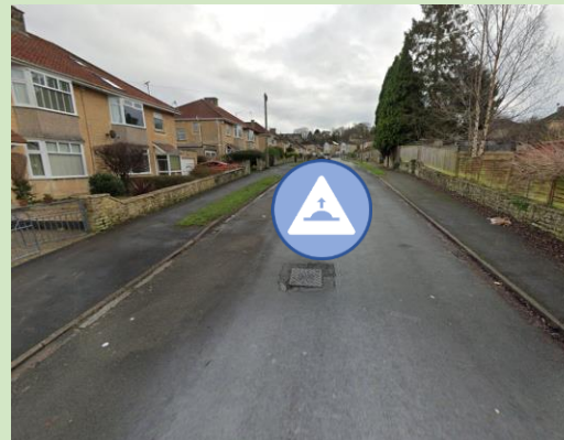
Traffic Calming along Egerton Road © Google maps 2022
