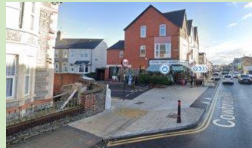
Continuous Crossing in Cardiff, Wales © Google Maps 2022
