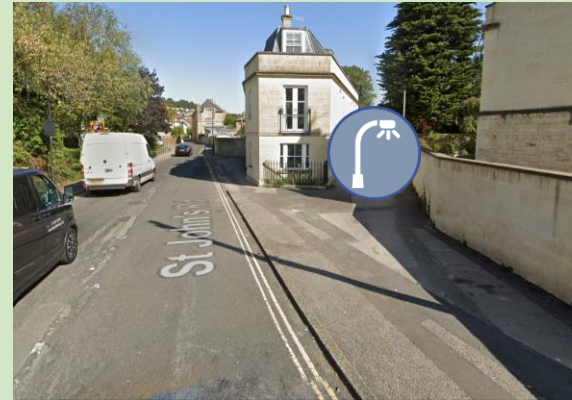
Footway in need of lighting improvements © Google Maps 2022
