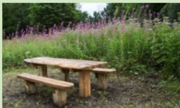
Rural picnic bench installation - © Cornford Creative
