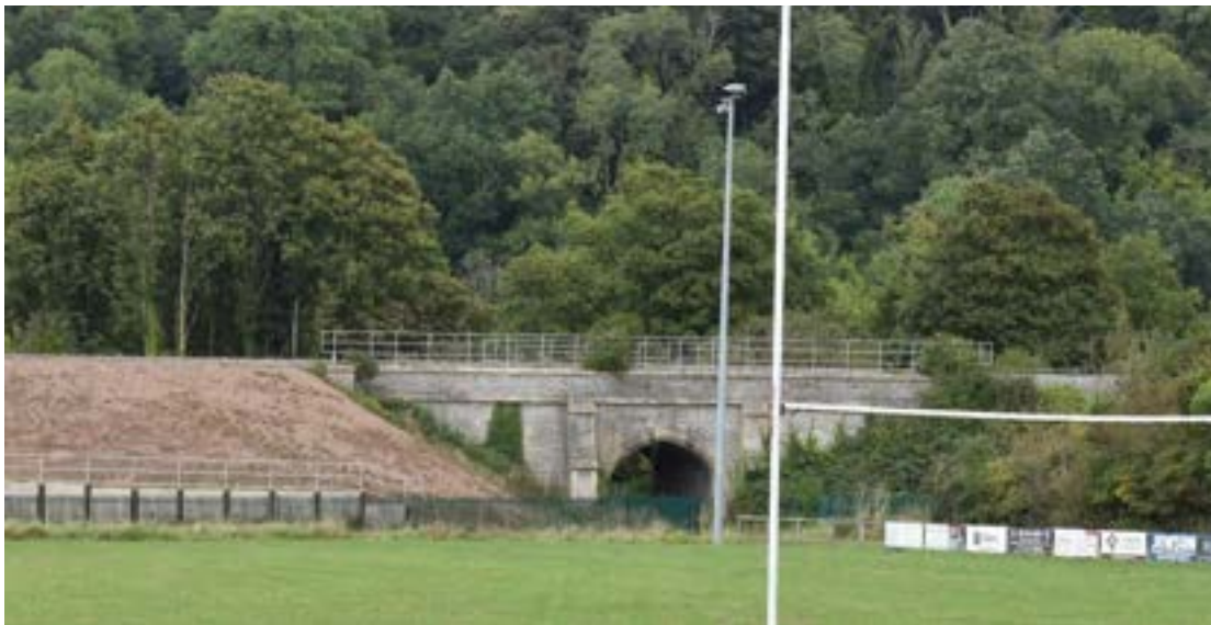
Figure 1.13: Stone Wharf Bridge
