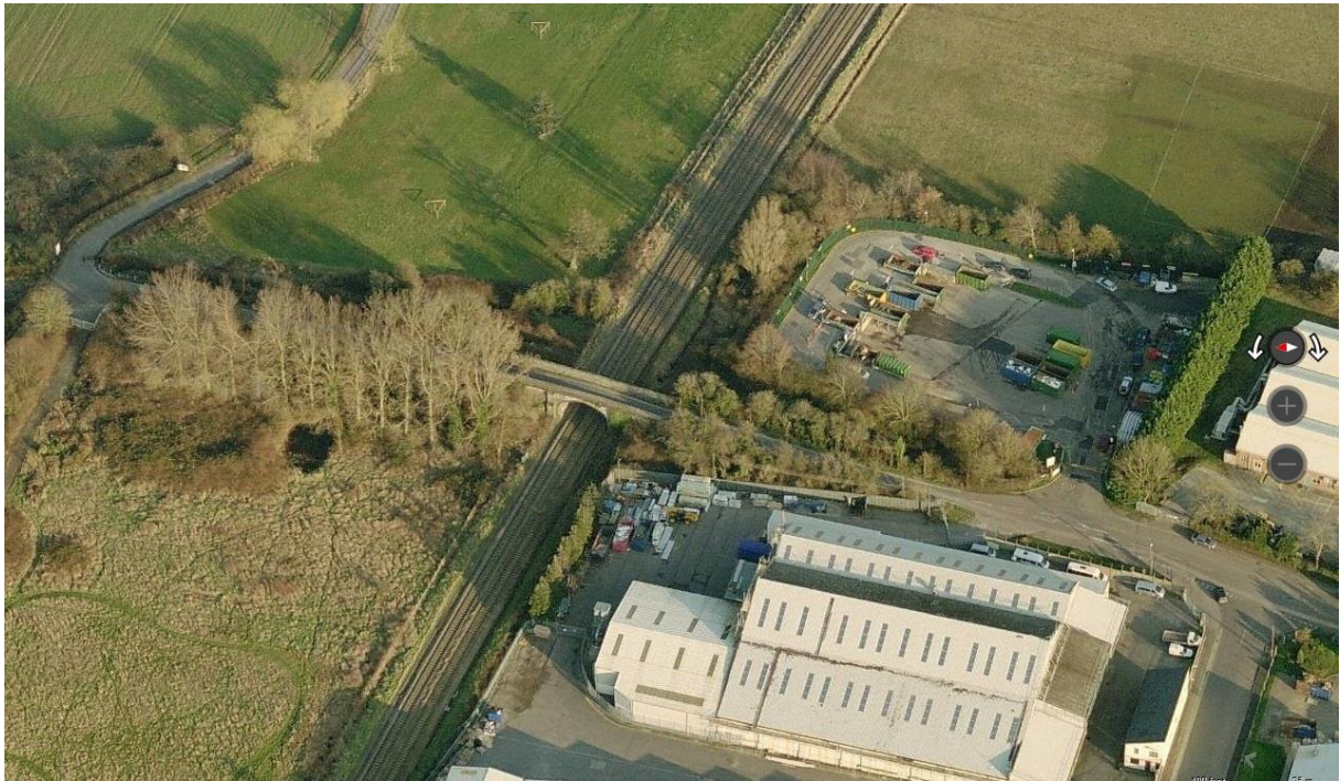
Figure 4.5: Pixash Lane Bridge aerial view from the west showing refuse depot
