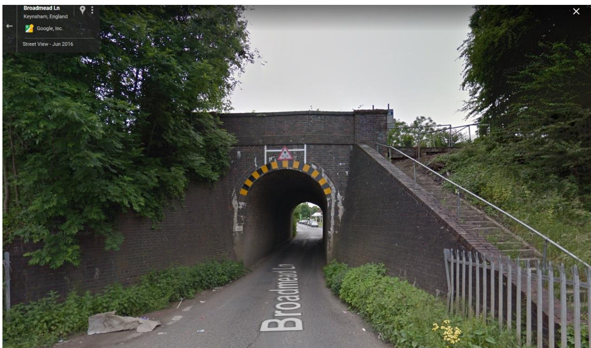
Figure 3.2: Broadmead Lane Bridge viewed from the north
