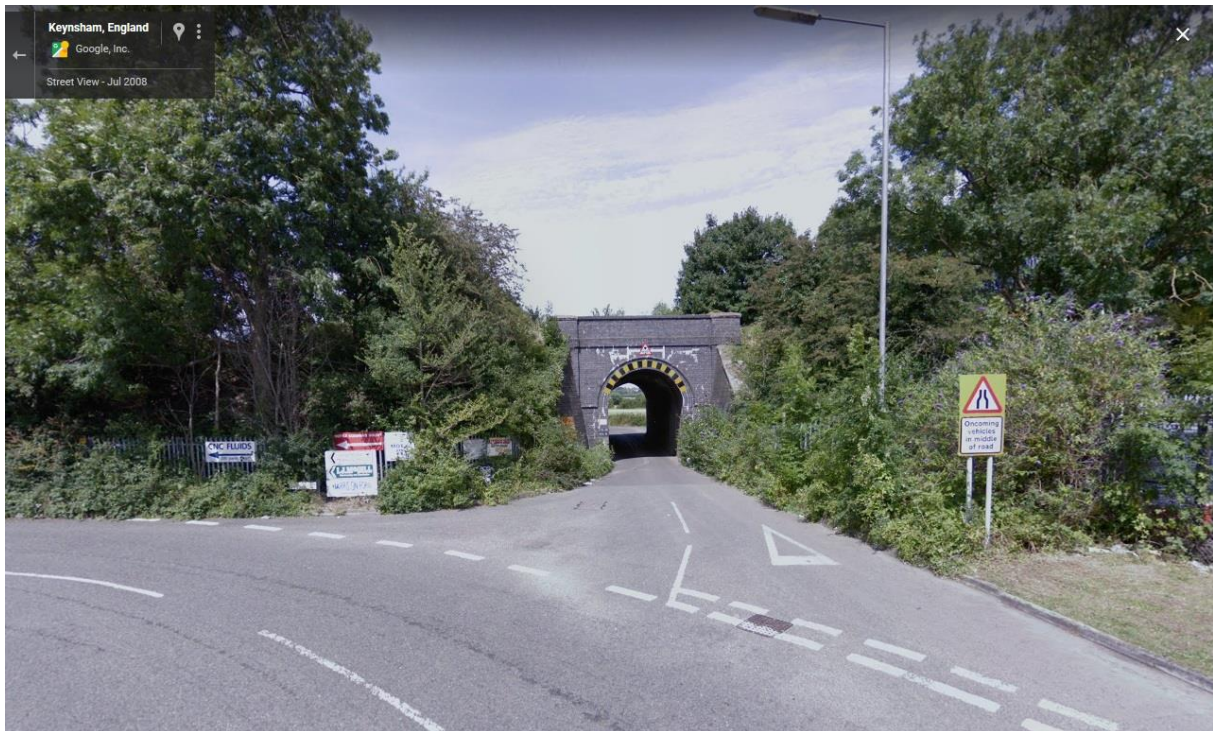
Figure 3.1: Broadmead Lane Bridge viewed from the south
